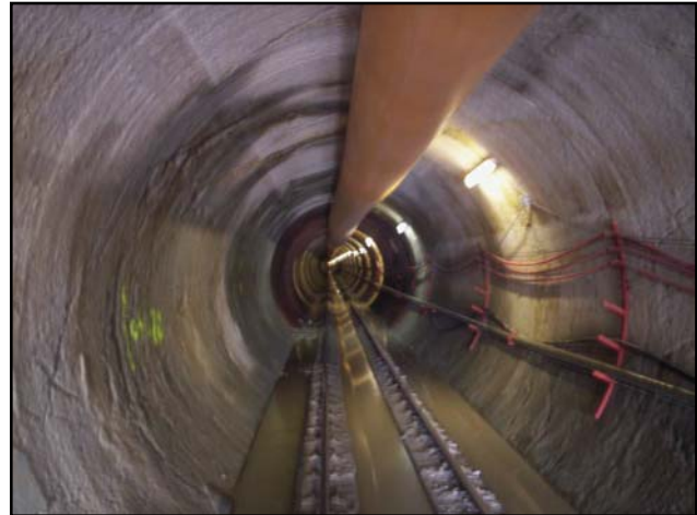
Figure N° 7. Excavation tunnel section.
